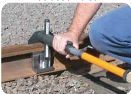
3. Select the location & check railhead wear
