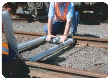
4. Positioning the PTW into the track
